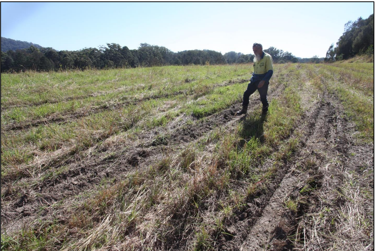
Figure 17: Inspection of the main access track along the ridge line- looking north
