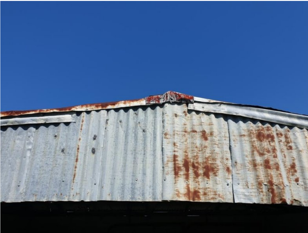
Photograph 7. Shed roof construction.
